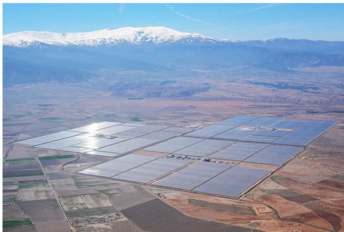
The Andasol solar power station in Spain.
