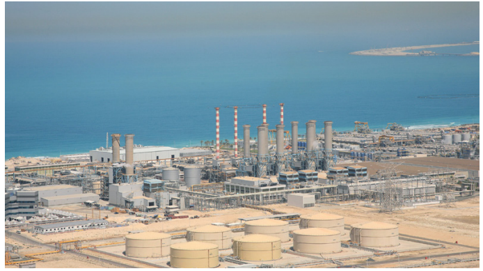
Desalination plants remove salt from naturally salty water, usually via distillation or reverse osmosis.
