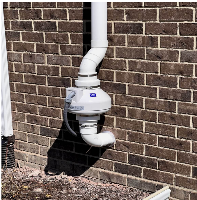
A radon mitigation system. Although airborne radon is responsible for the vast majority of radon-caused cancer deaths, the EPA only has authority to regulate radon in drinking water, so it is up to individuals to assess their risk and consider means of mitigating it.
